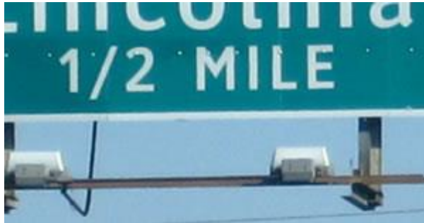
Figure 5a. NOT ACCEPTABLE: Incorrect alignment of fraction numerals and inadequate interline and edge spacing.
