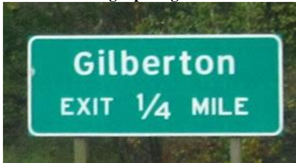
Figure 5b. ACCEPTABLE: Correct alignment of fraction numerals.
