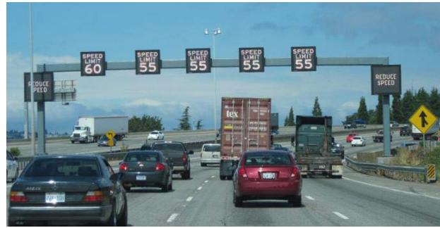
Figure 1. A sign bridge over Northbound I-5 cautioning drivers of adverse conditions ahead.
