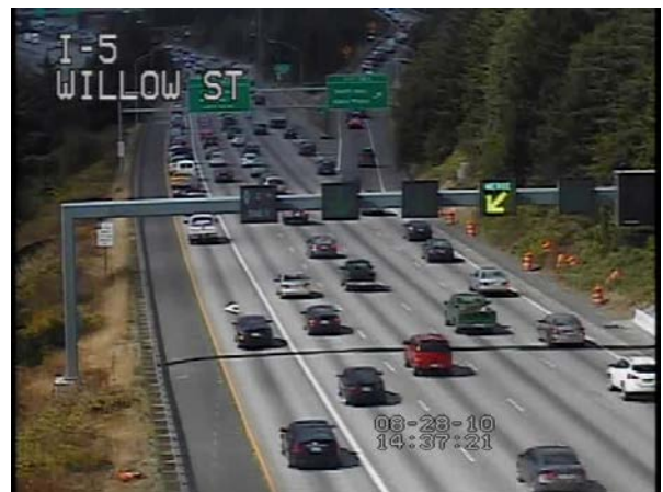
Figure 4: A merge arrow indicating the right center lane is blocked ahead.
