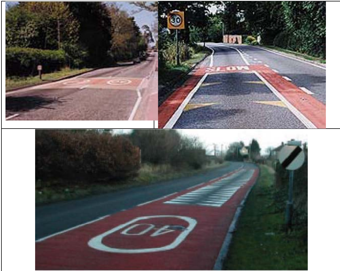
Figure 3: Red Markings with Posted Speed Limit Signs Used in European Gateways (image source: Sustrans, 2004)
