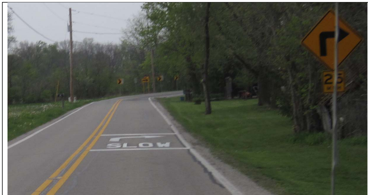
Figure 4: Use of the on-pavement advance curve marking in Ohio
